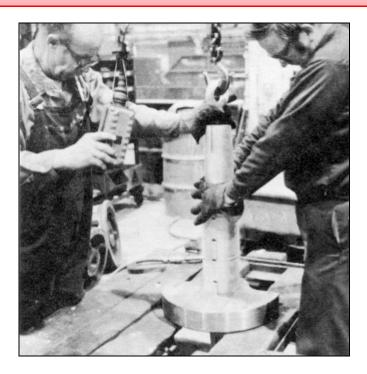
Figure 4.5 Arrangement for assembling counterweight on shaft.
